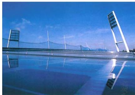
Roof of Bremer Weser Stadium
